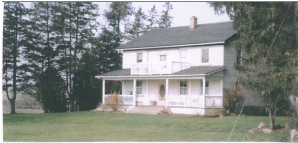
Brick house built on Lot 19 NSR by Christian Gascho in 1856
